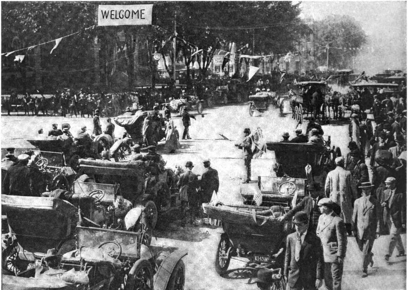
Scene in Crown Point's Courthouse Square, Which Was a Storm Center, with Fakira in Abundance
